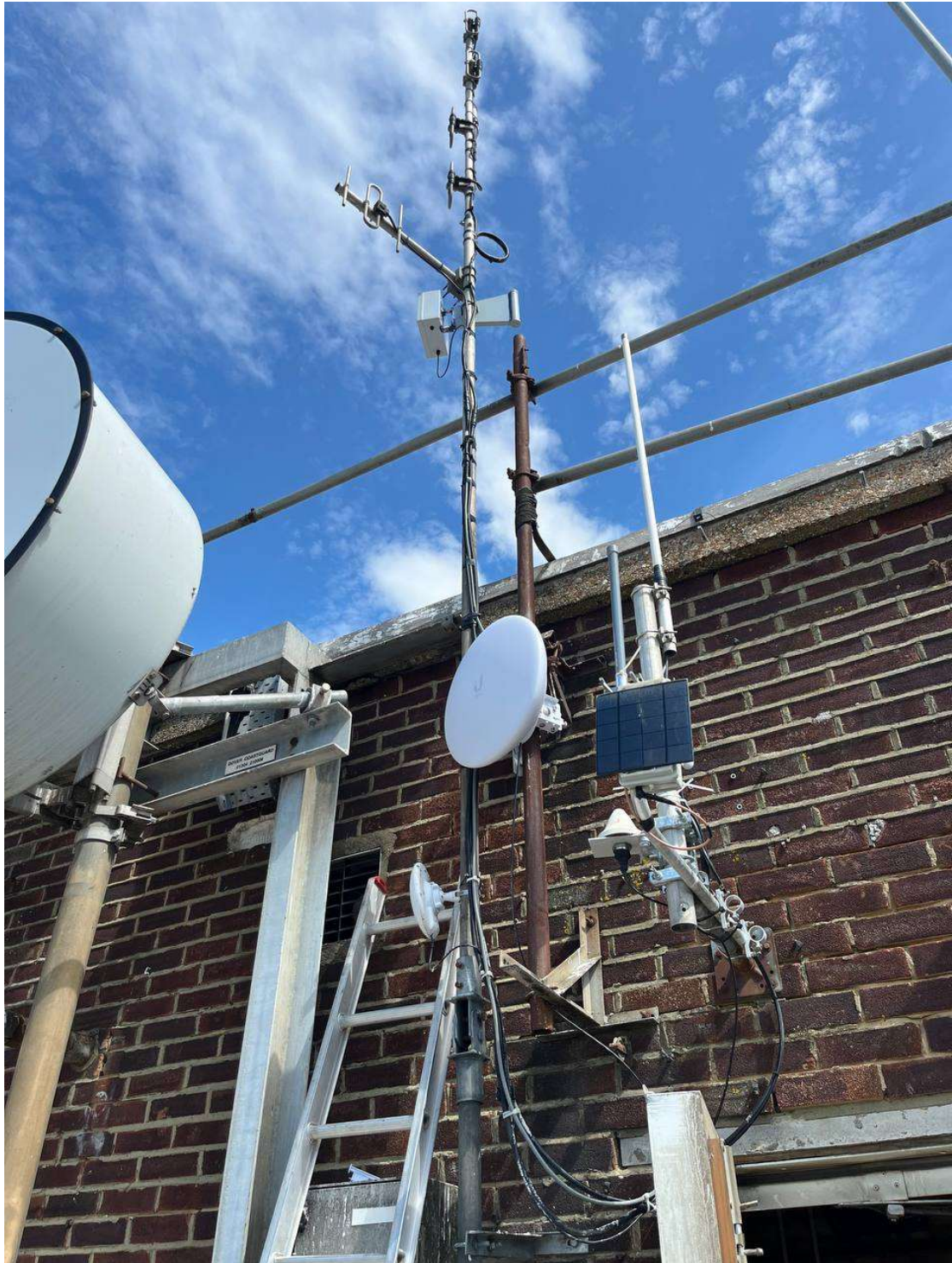
Figure 6 The outdoor unit just below the 3element 70cm Yagi
